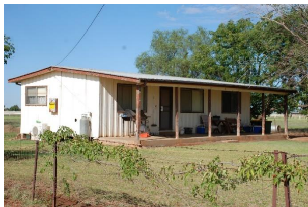
Plate 26: Former Caretaker's Cottage
