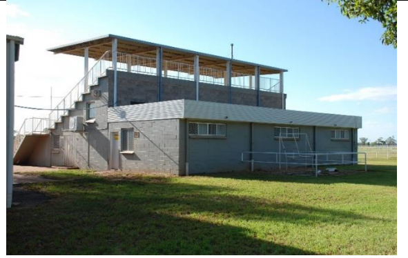
Plate 20: Rear of brick grandstand
